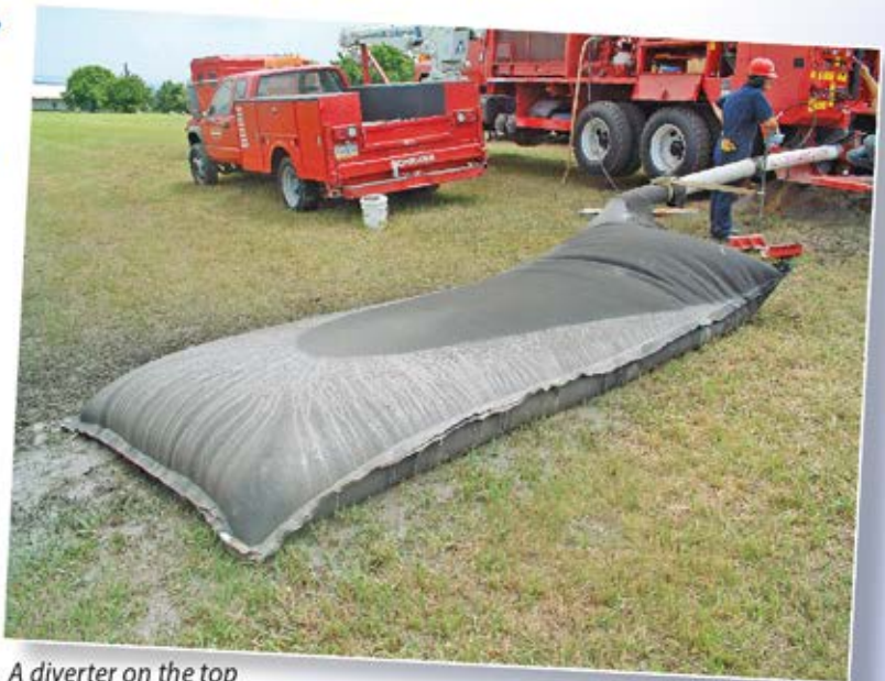
A diverter on the top of the well casing is sending 30 gpm of groundwater and drill cuttings and 1,200 cfm of air through the blooie pipe into the sediment filter bag for treatment.
