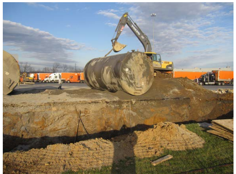
Schneider National, Inc. UST Removal and Installation – Carlisle, Pennsylvania
