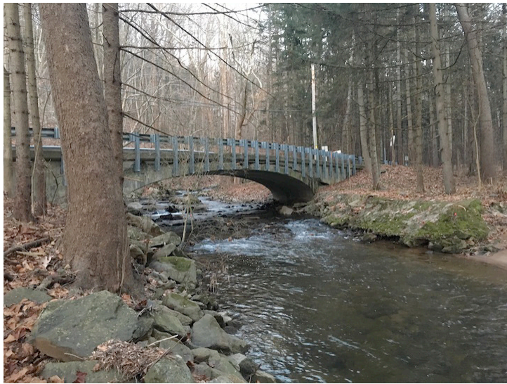
Single span bridge replacement in alluvium.
