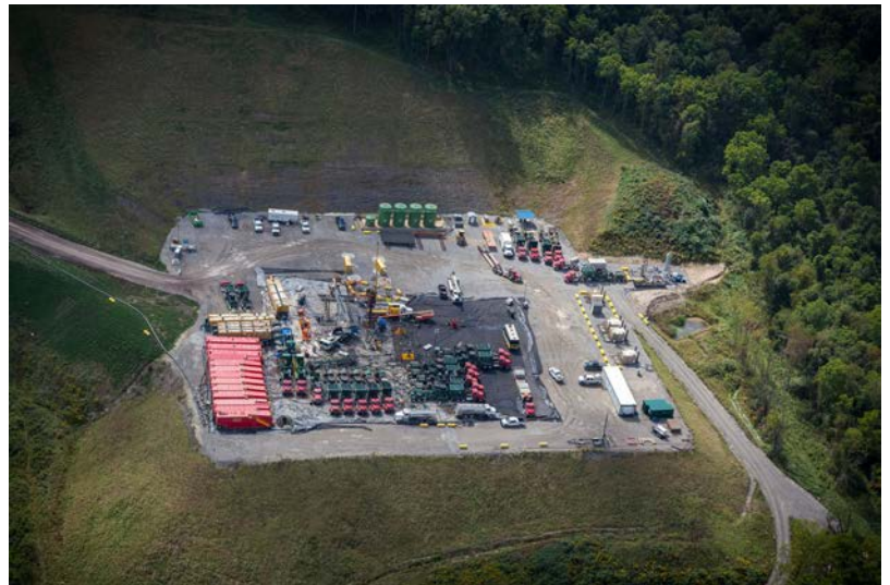
Marcellus Shale hydraulic fracture treatment, Western PA. The liner under all the equipment would contain any accidental spills so the groundwater won't be impacted.
